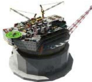
Figure 3.5: Mono-column floater
