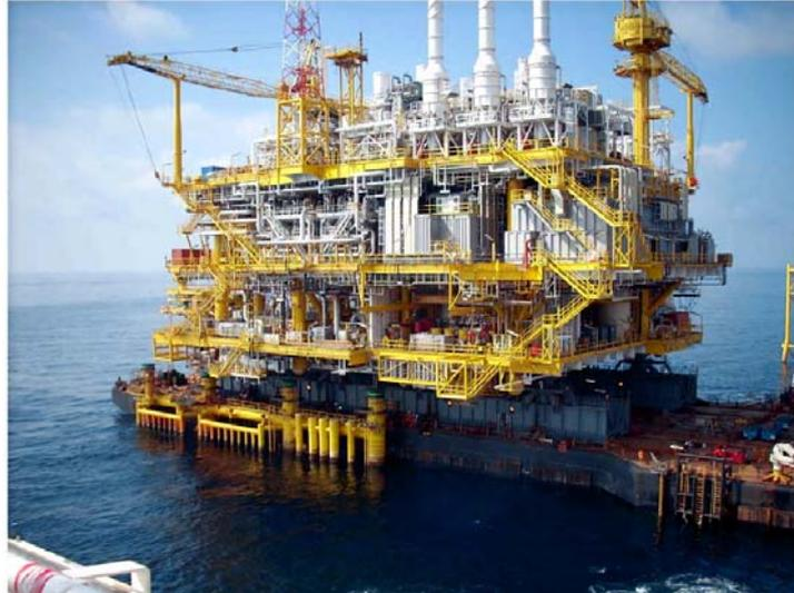
Figure 5.3: Arthit Deck – as the barge enters the jacket slot
